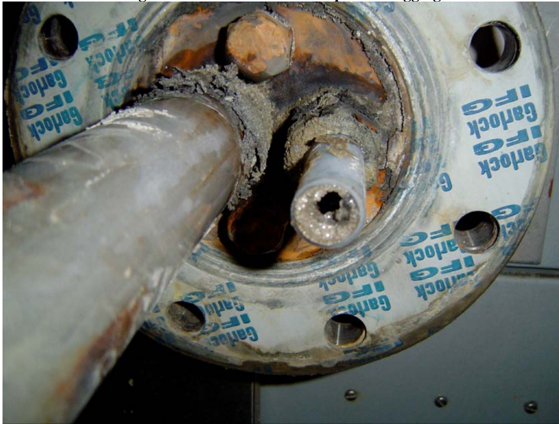
Figure 13 – Inertial Probe Loop Exit Plugging
